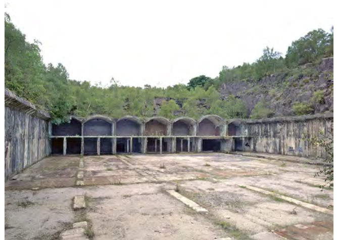
Llanberis Pits Site 1 showing the cleared area with the surviving galleries beyond. Photo Nick Catford
